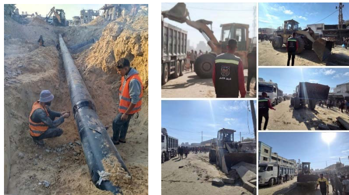
Right: Khan Yunis municipal teams clearing debris to reopen roads (Alaa al-Bitta's Facebook page, October 13, 2025). Left: Municipal teams repairing the sewage network (Khan Yunis Municipality Facebook page, October 20, 2025)
