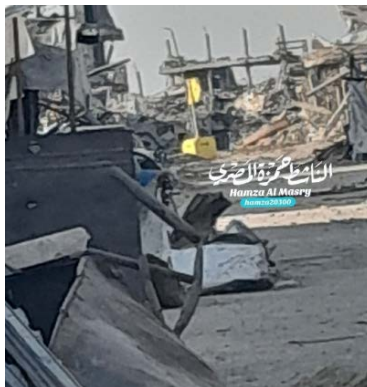
A new yellow concrete block near the vegetable market in the al-Shuja'iyya neighborhood (Telegram channel of Hamza al-Masri, November 21, 2025)
