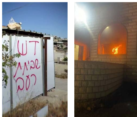
The fire at the mosque in the village of Tuwani and the graffiti on buildings (Al Jazeera Palestine Telegram channel, July 19, 2026)
